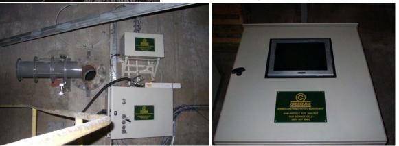
The development was customer driven, with a requirement for an improvement over optical type opacity stack measurements which, work satisfactory for opacity when the particulates remain small and unchanged, however, their sensitivity is impaired when the particle size distribution changes in the flue gas. A simply analogy is comparing water mist to rain, where the opacity reduces but total particulate mass increases - Reflectance of light proportional to 1/ diameter of particles.
