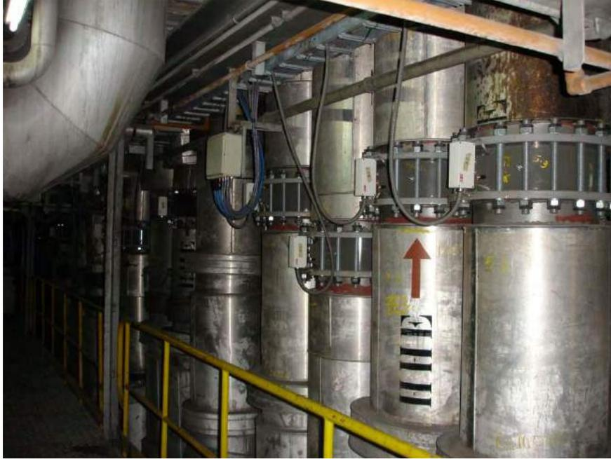
**Photo 1 - PfMaster a triboelectric Coal Flow monitoring sensors**
