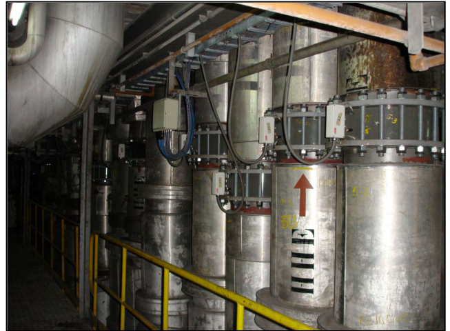
PfMaster Installed In Vertical PF Lines:
