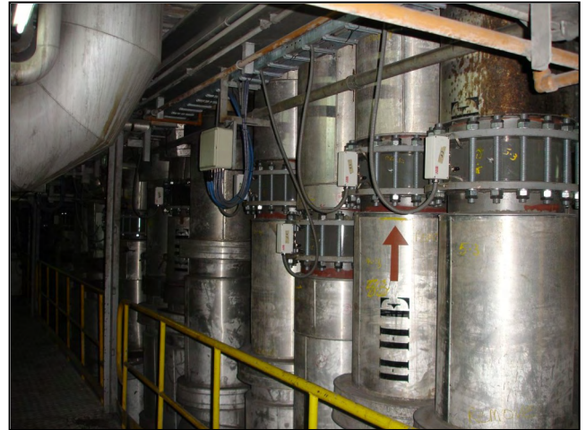
PfMaster Installed In Vertical PF Lines:
