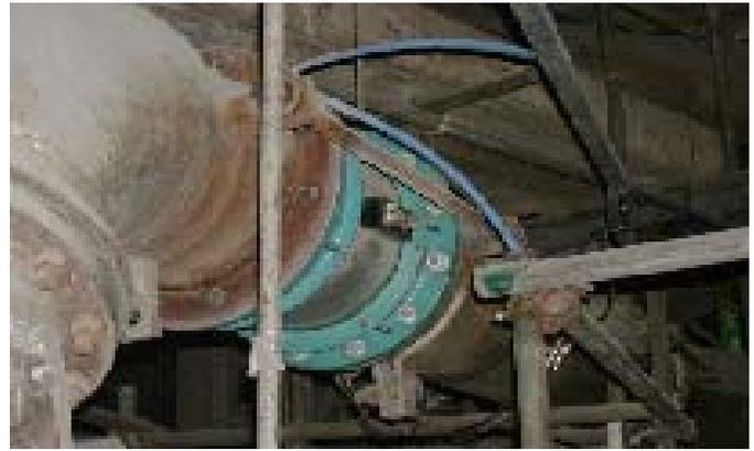
The sensor, being a spool-piece, provides the highest performance in the presence of roping / mal-distribution of pf.
