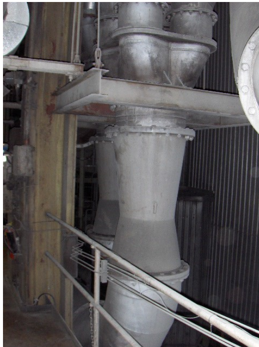
Figure 1: Original Arrangement of Nanticoke PF Distributor
