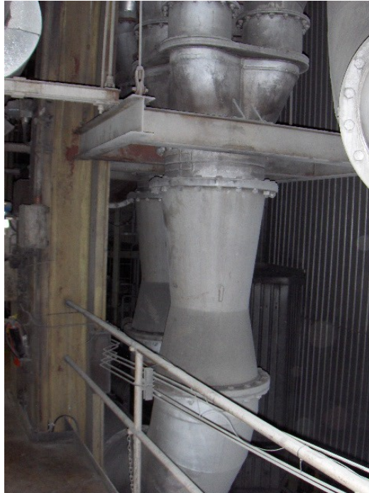
Figure 1: Original Arrangement of Nanticoke PF Distributor
